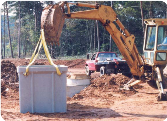
Lift and position enclosure with backhoe.
