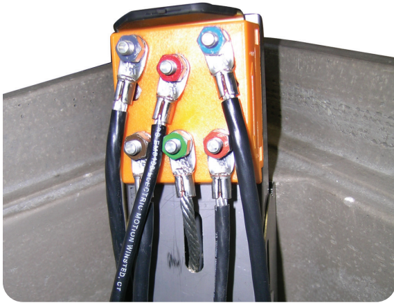
Bonding Harness Or Locate Wires
