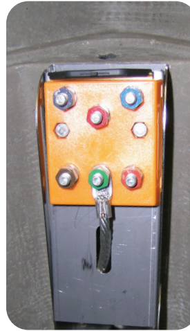
Test Station or Isolation Switch
