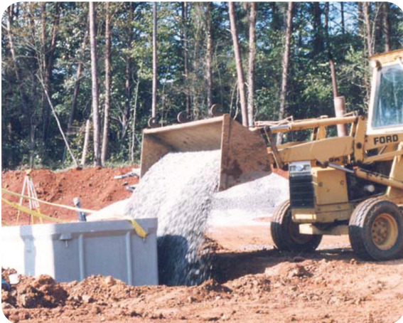
Place gravel in the enclosure and around the side. Lift enclosure to let gravel run underneath.
